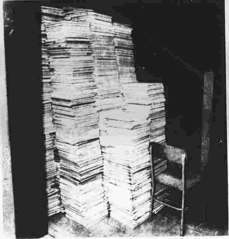
Stacks of ceiling tiles clutter a stairwell at Manchester High School. As soon as fire door wiring in the corridor ceilings can be completed, these tiles will be used to patch up the gaping holes in those ceilings now.
